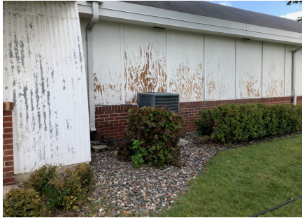
Before: West side of Quonset building after it was power washed and scraped, and before it was painted.
