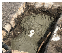
Cement was poured on top of the repaired pipe to keep the pipe from being crushed in the future.
