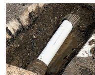
New pipe installed. Vinyl collars were placed over each end to close any gaps.
