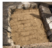
Sand was packed down on top of the cement.
